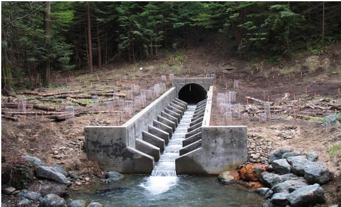
*Chadd Creek (D1) Fish Passage structure
