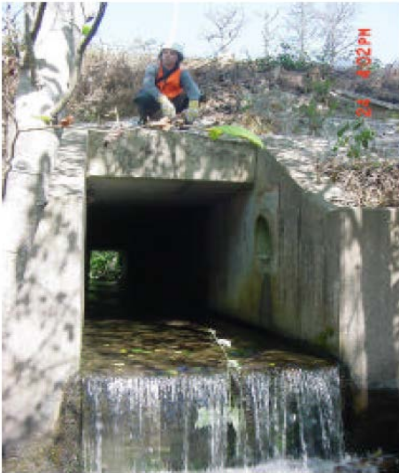
Culvert outlet
